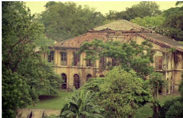
A dilapidated Suffolk House before restoration
